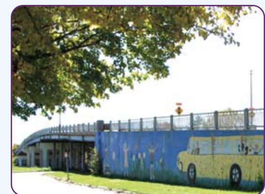
Hamline Avenue where it crosses over Ayd Mill Road
